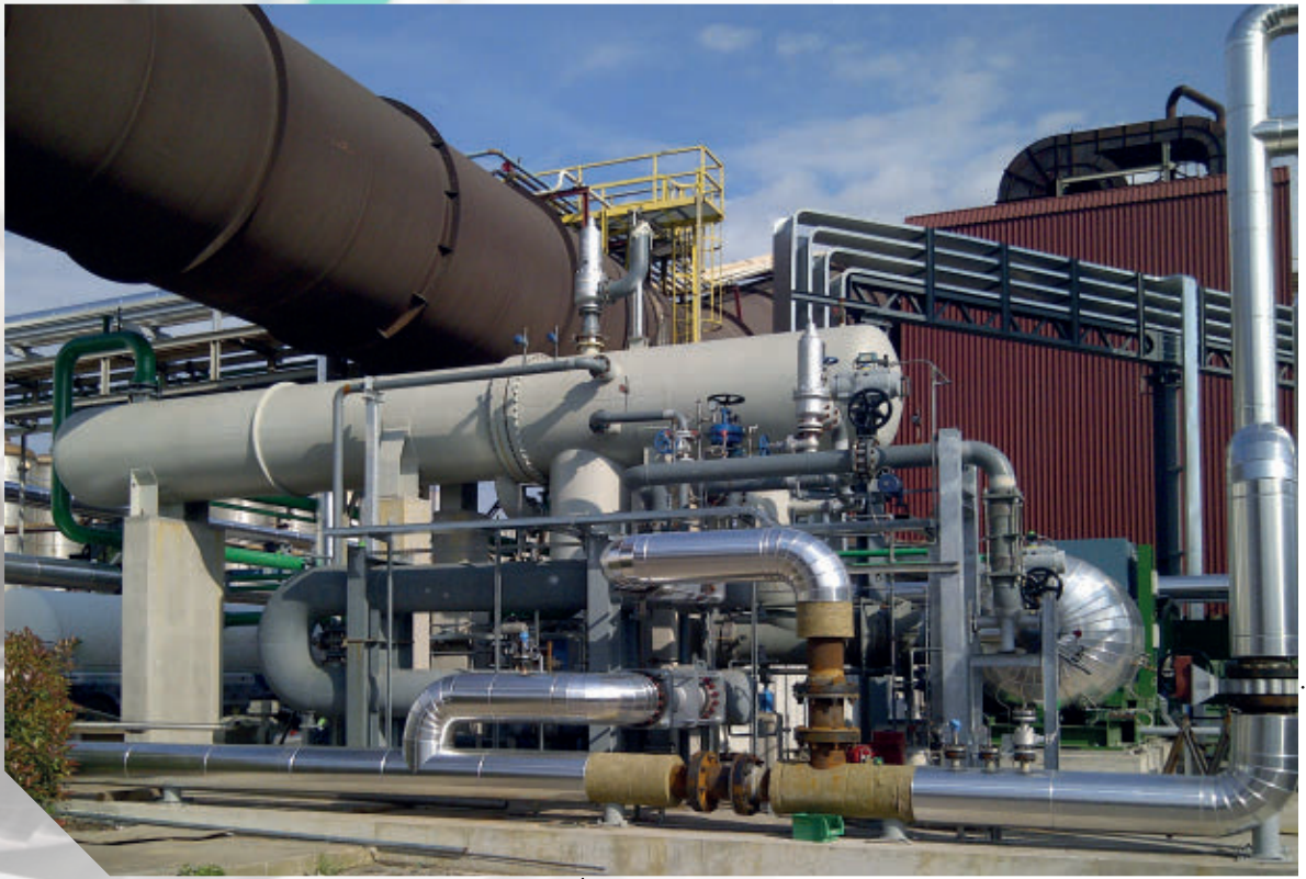
An Organic Rankine Cycle (ORC) installation by Italian specialist Exergy for waste heat recovery.
